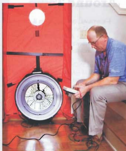
Jim Clark of ESS conducts a blower door test during home energy audit
